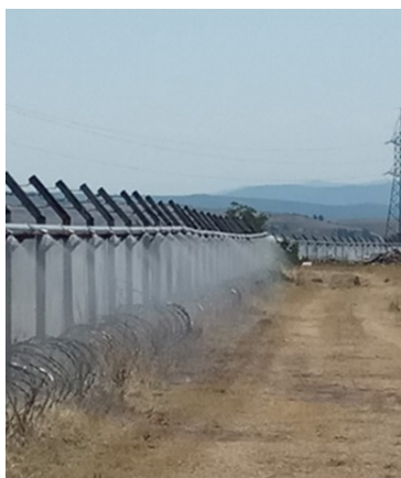
Figure 8. Water curtain system adjacent to the railway
